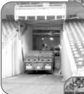
Stadium Access Lift
