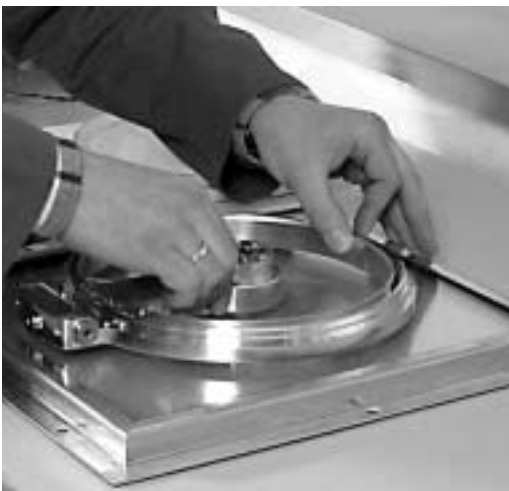
Installation and bonding of the VISIPOINT
